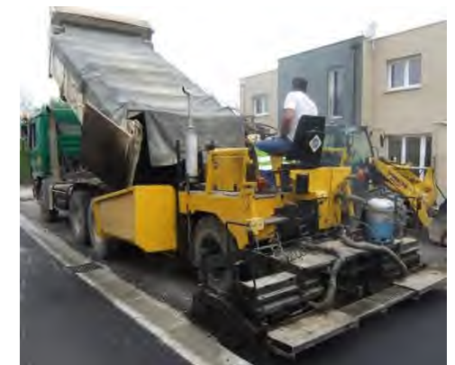
Figure 102 - Finisseur (source: Gillet TP)
